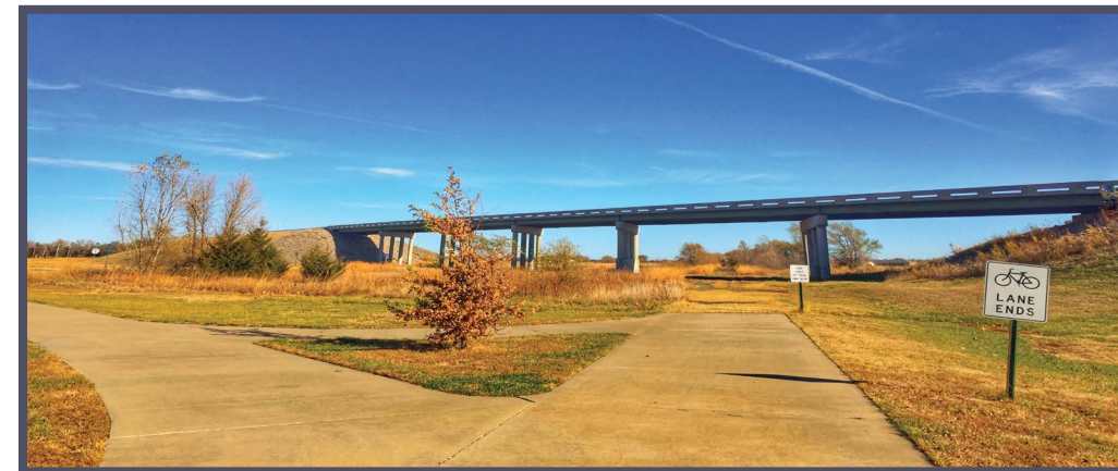
The picture to the left shows where the next phase of the trail will begin.
